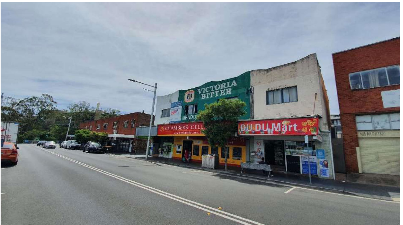
Figure 3: Retail buildings on the western side of the site fronting Railway Road.
