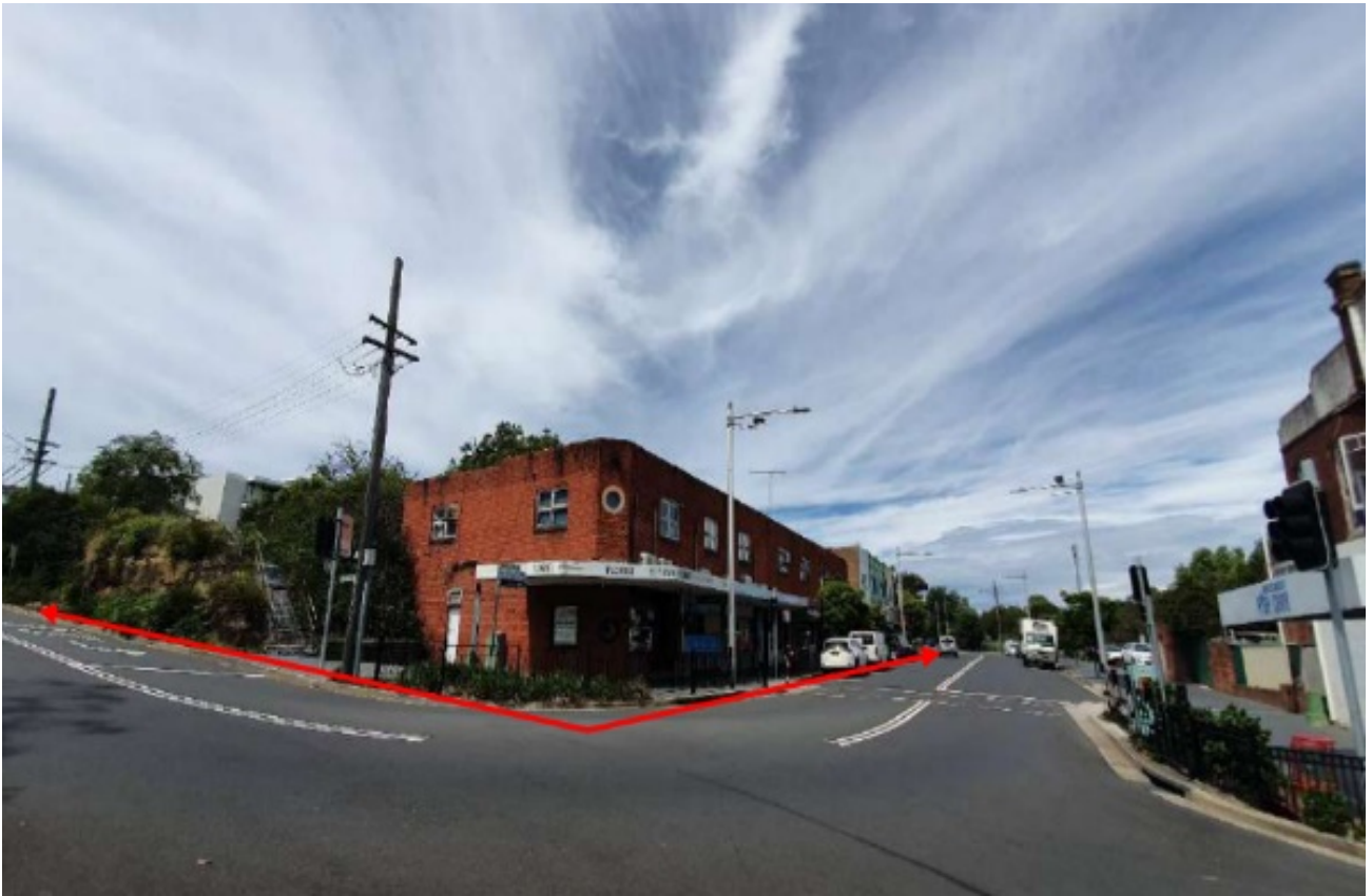
Figure 2: Existing retail building on the northwest corner of the site, on the intersection of Railway and Constitution Road. (Red line denote the development site).
