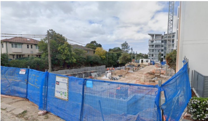
Figure 9: LDA 2015/540 currently under construction, part 5/part 6 RFB, located opposite in Faraday Lane (and facing Constitution Road).
