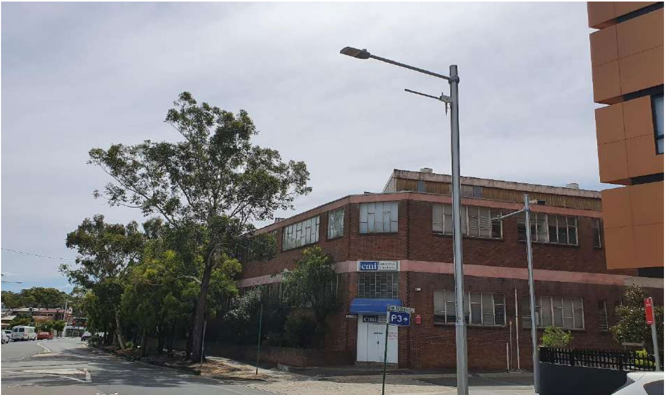
Figure 4: Southwest corner of the site on the intersection of Railway Road and Underdale Lane.
