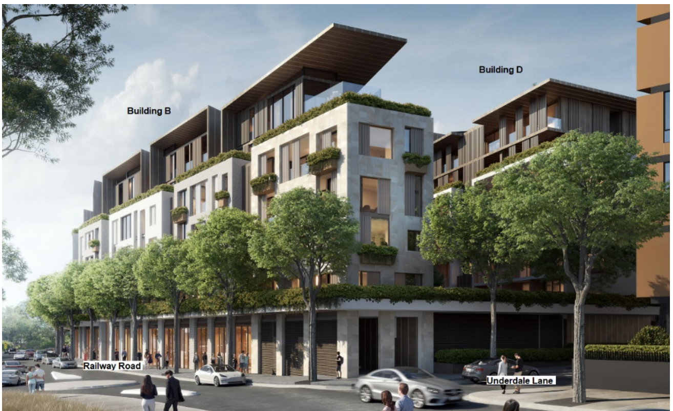
Figure 17: Photomontage of the development as viewed from Railway Road near the intersection of Underdale Lane, Buildings B & D are shown.
