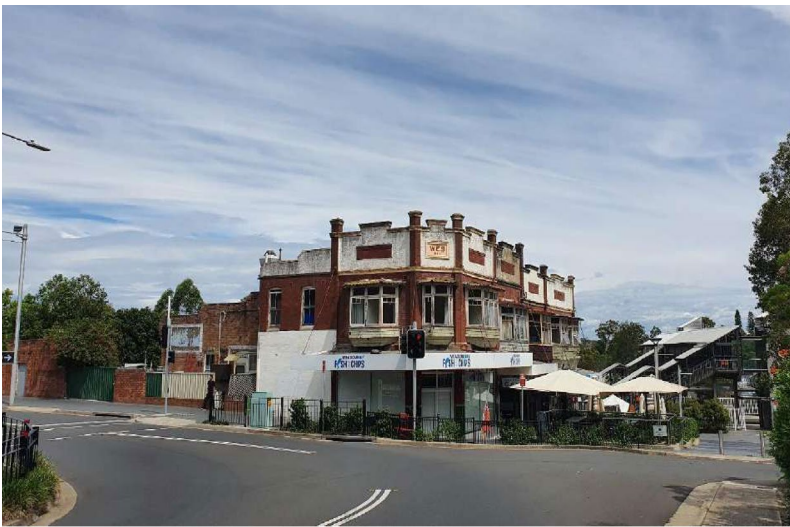
Figure 12: Directly opposite at 58 to 64 Constitution Road, 2 storey heritage item and adjacent Meadowbank Station.
